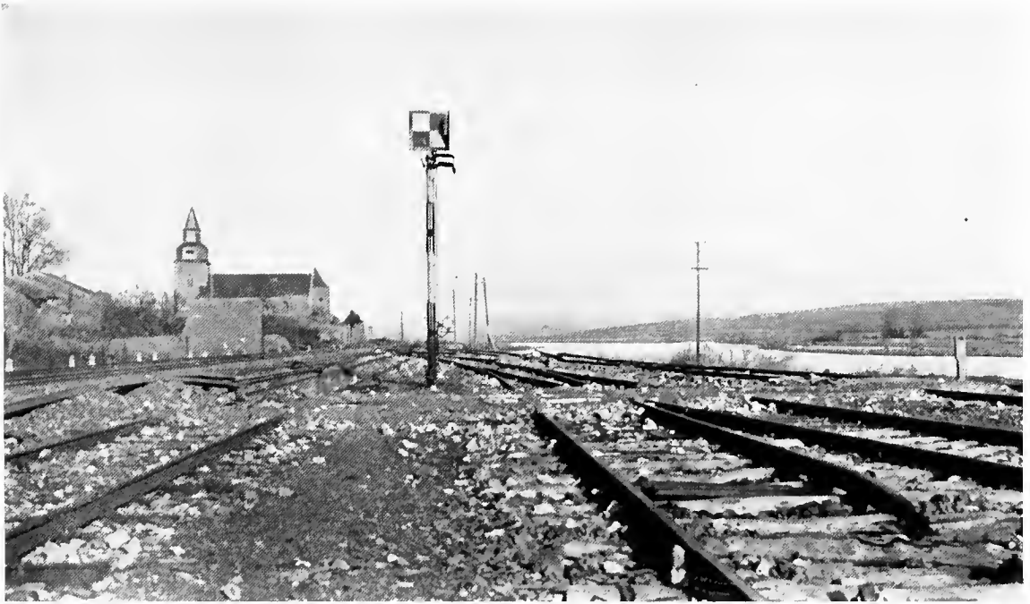
Villers Devant Mouzon, Point where Bridge was Constructed Across the Meuse by the 77th Division—Looking North
