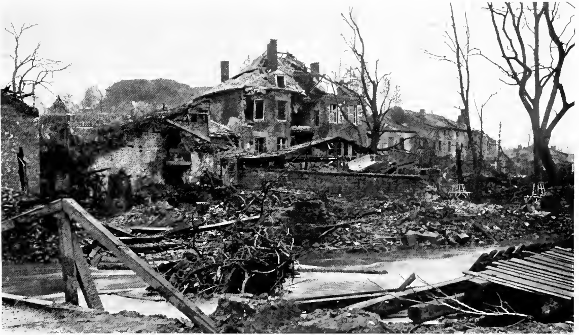
Ruins of Grand-Pre, Looking North
