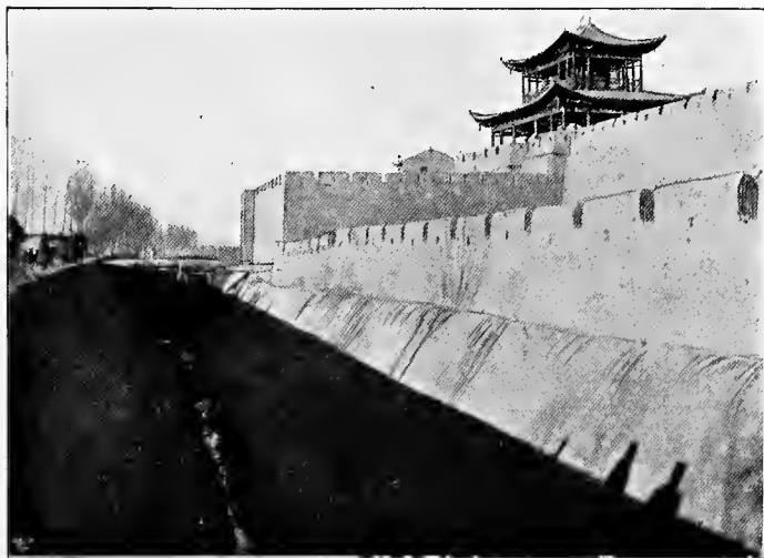
THE WALL OF YANGI SHAHR, YARKAND.
