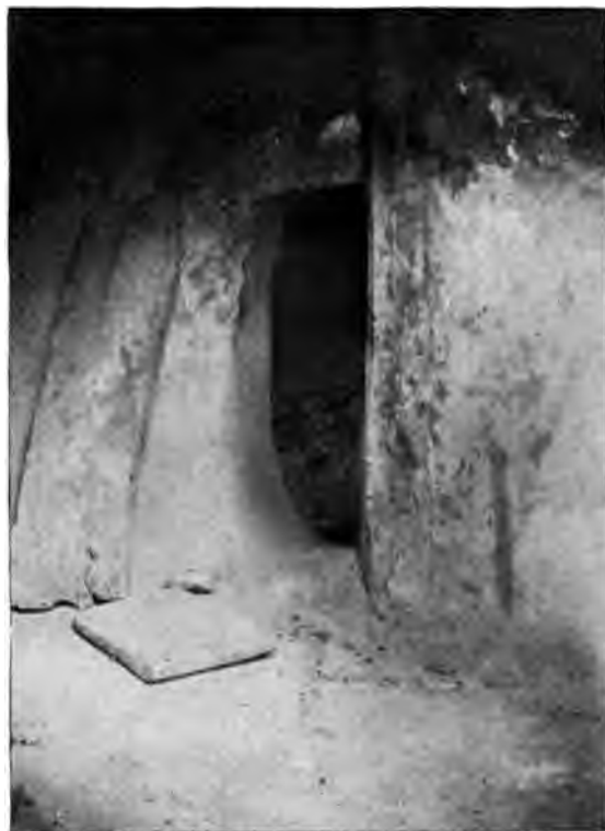
INTERIOR OF TEMPLE OF AIRI DEO. DÖL, KAMAON.
